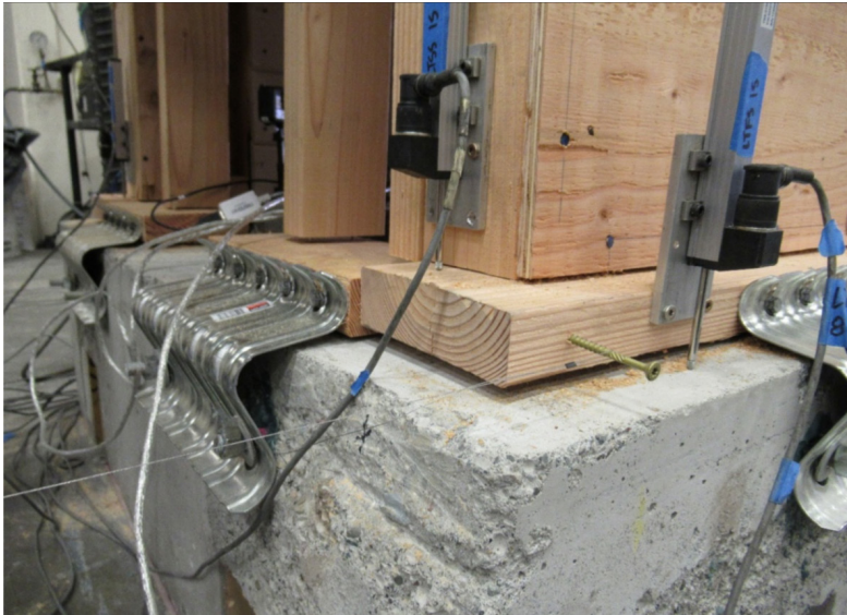
Figure 2.3. Foundation sill plate uplift during full scale testing; source: Figure 4-20 from Large-Component Seismic Testing for Existing and Retrofitted Single-Family Wood-Frame Dwellings
