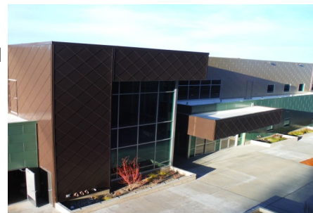
Jackson County's new Health & Human Services Building
