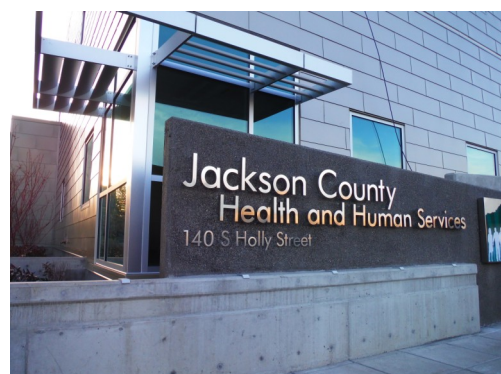
Jackson County's new Health & Human Services Building
