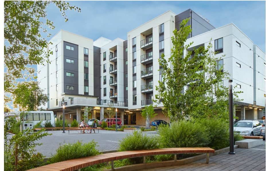
Gilman Court in Portland includes 60 homes in this LEED certified Homes for Mid-Rise Gold status.
