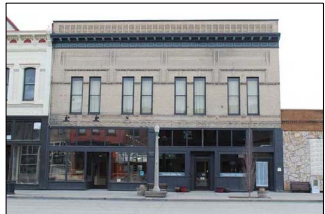
Haskel Building After Rehabilitation:
