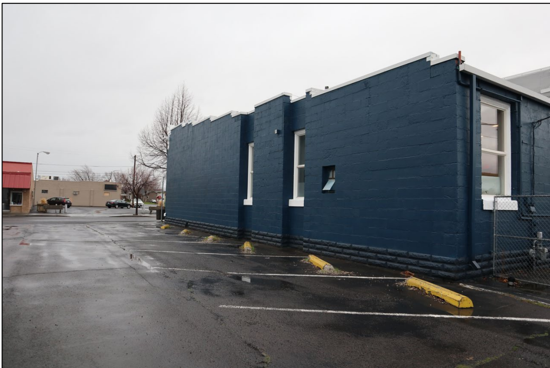
Photo 4 of 19. North elevation, camera facing southeast.
