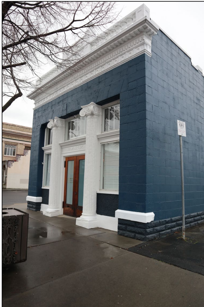
Photo 12 of 19. East façade, camera facing southwest.
