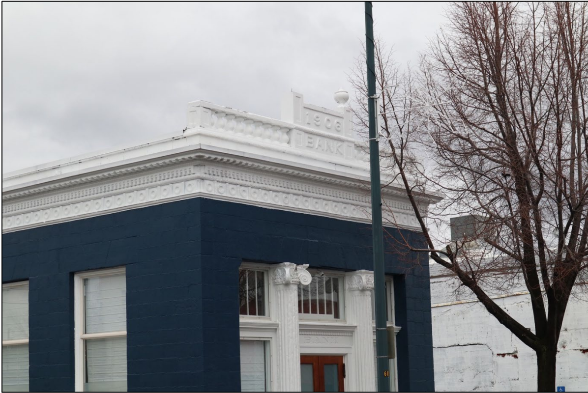
Photo 17 of 19. East façade balustrade detail, camera facing northwest.
