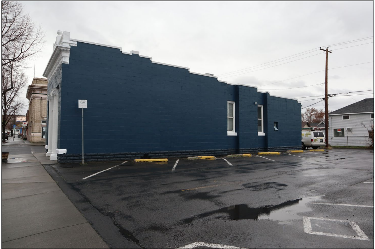
Photo 5 of 19. North elevation, camera facing south.
