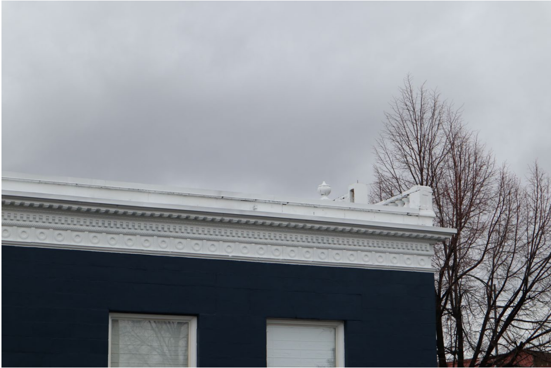
Photo 11 of 19. Entablature detail on south elevation, camera facing north.
