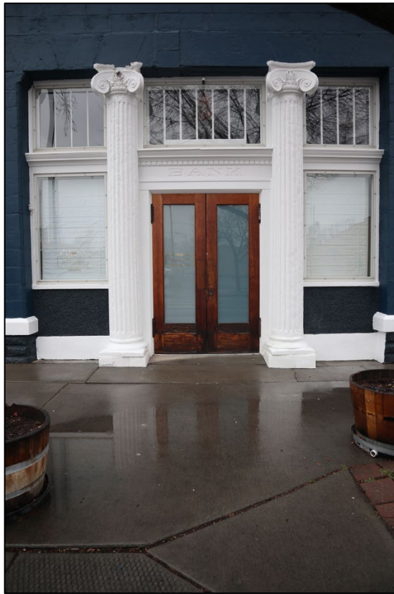
Photo 13 of 19. East façade and primary entrance, camera facing west.
