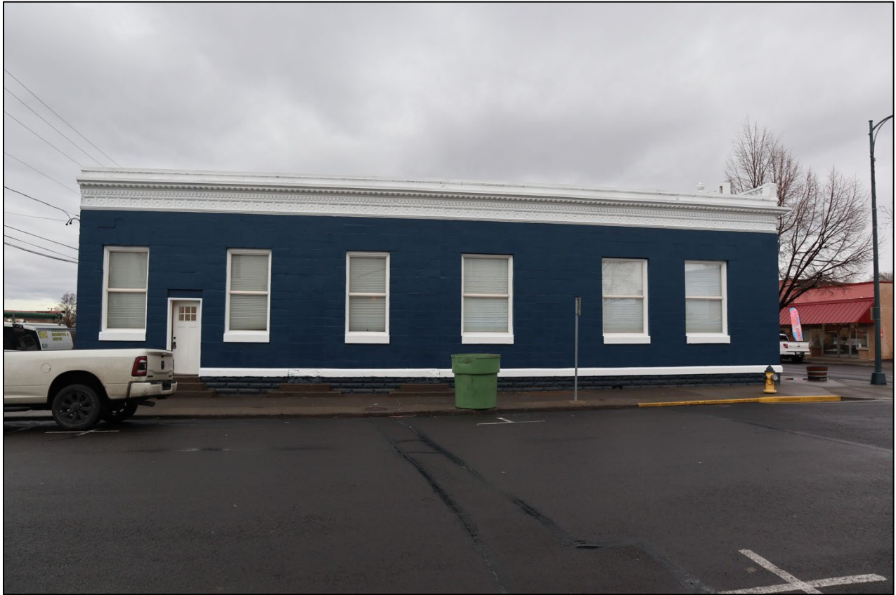
Photo 7 of 19. South elevation, camera facing north.
