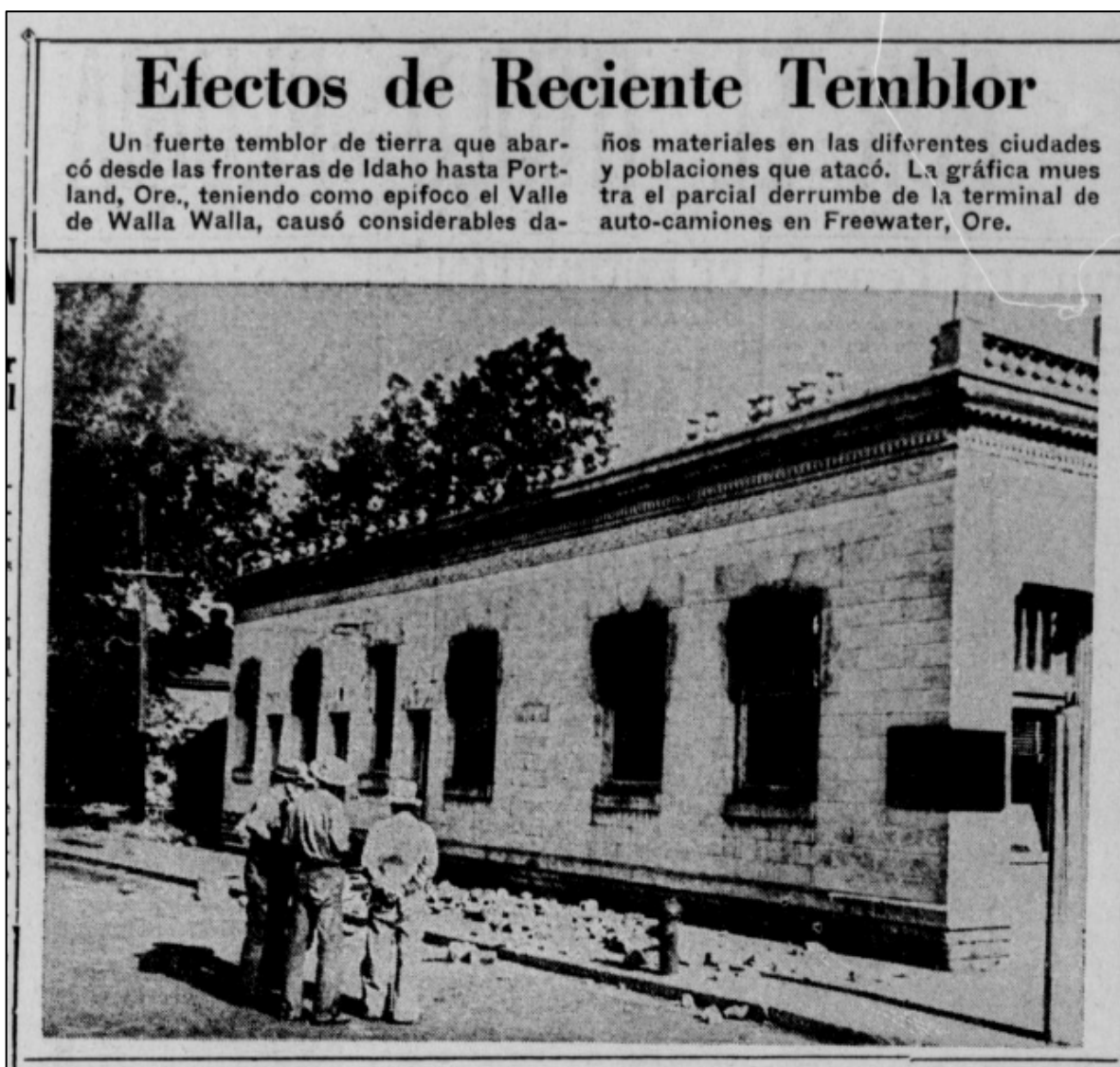
Figure 8. Historic photo from La Opinion (1936). Headline translates to “Effects of Recent Earthquake.” Text reads: “A strong earthquake that spanned the borders of Idaho to Portland, Oregon, with the Walla Walla Valley as its epifocus, caused considerable material damage in the different cities and towns it attacked. The graphic shows the partial collapse of the truck terminal in Freewater, Oregon.” (Image from page 8, La Opinion , July 21, 1936; translation courtesy of Google Translate.)
