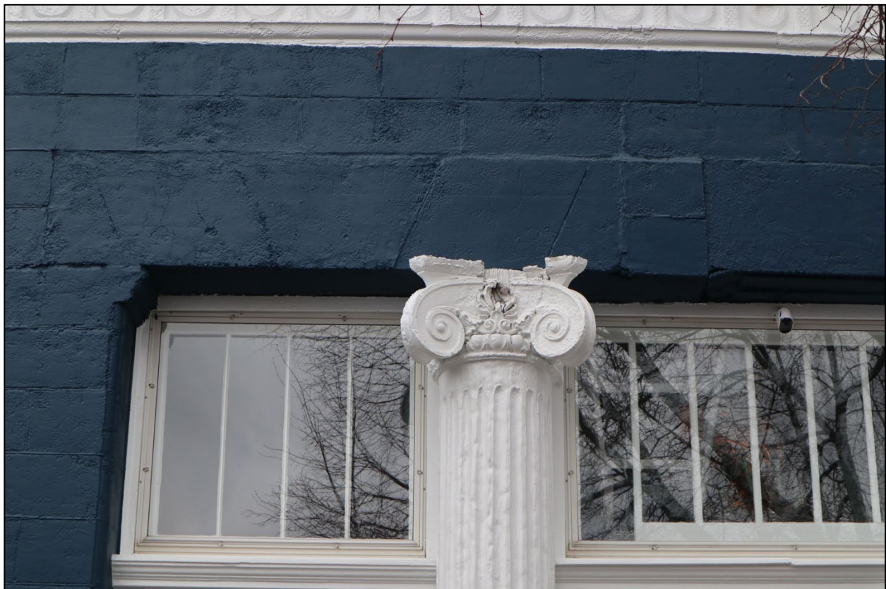
Photo 10 of 19. Column detail, camera facing west.
