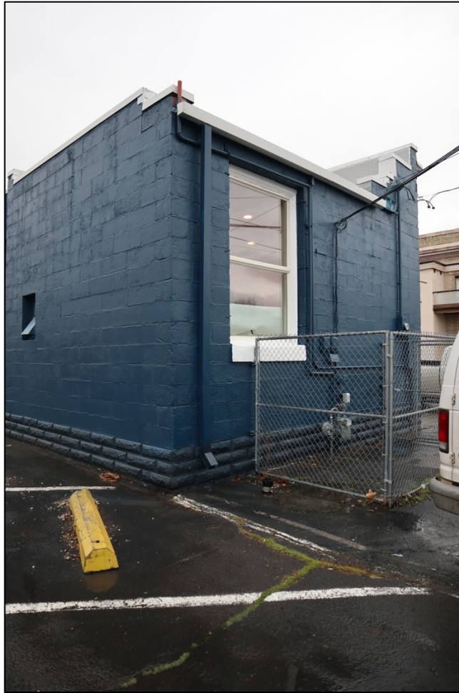
Photo 3 of 19. West elevation, camera facing southeast.
