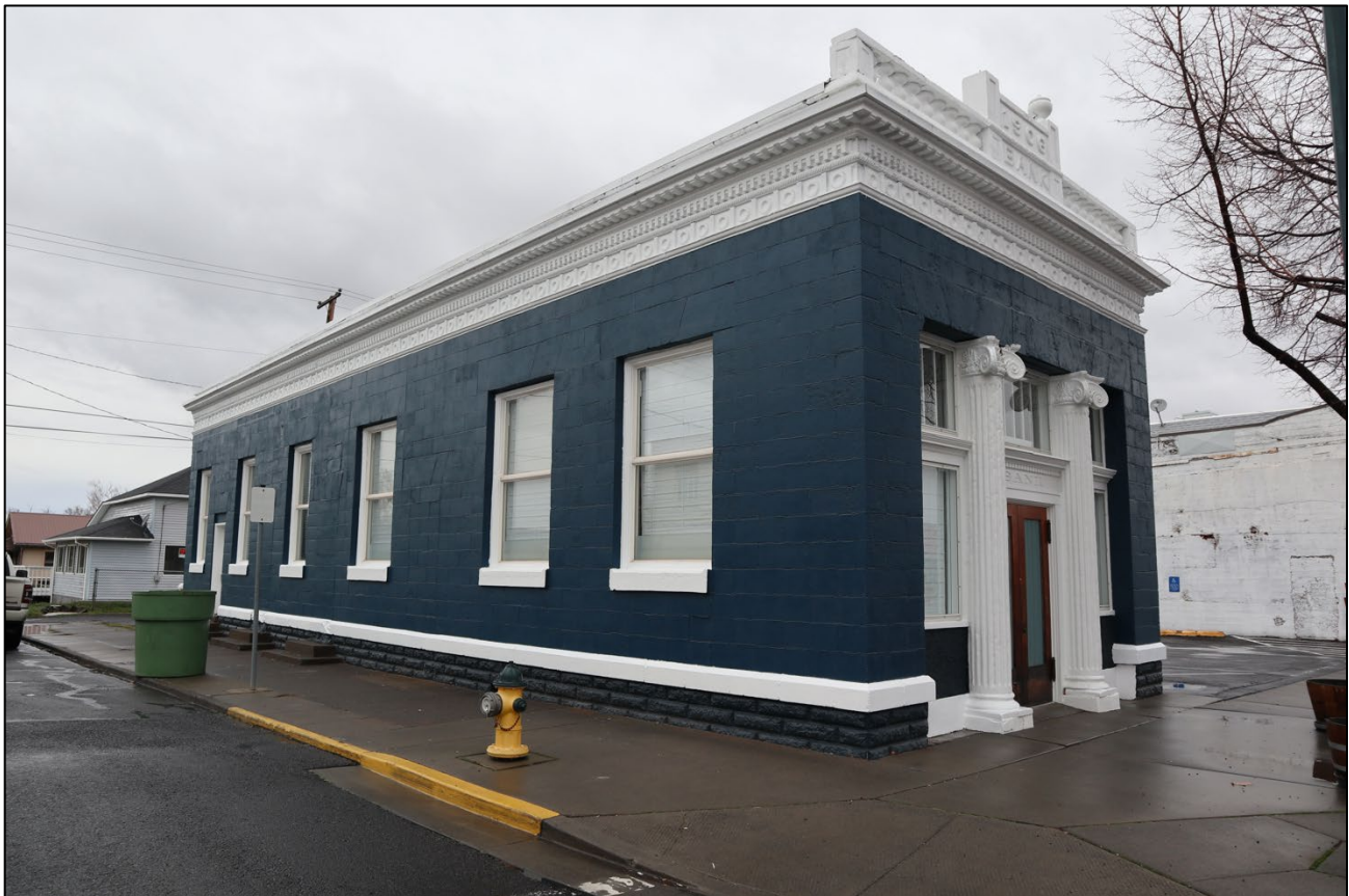
Photo 6 of 19. East façade and south elevation, camera facing northwest.
