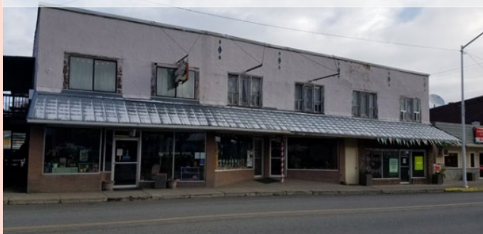
Weaver building before rehabilitation i
