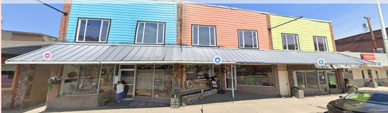
Weaver building today
