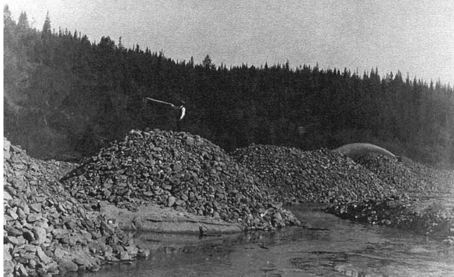
Figure 1.2.1 - Piles of boulders are left behind after hydraulic mining with the Ruble Rock Elevator. Photo taken on Coyote Creek circa 1900 (GCW)
