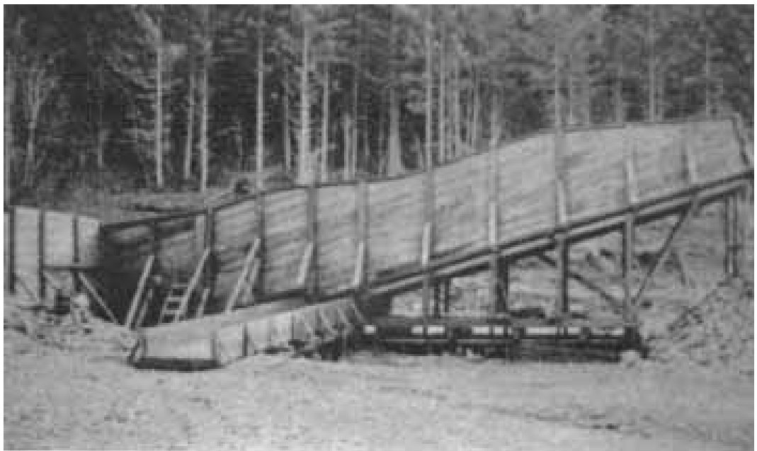
Figure 1.3.3 - The Ruble Rock Elevator was used to stack boulders and other hydraulic mine tailings while coarse gold was captured in the elevator’s lower sluice box. Photo, circa 1900 (GCW archives).
