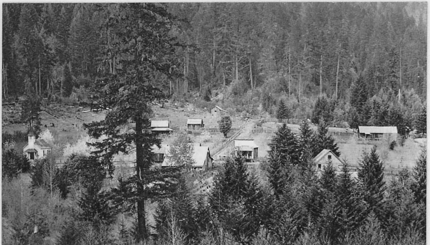
Figure 3.1.1 - Looking northward at Golden, circa 1905 (GCW archives). Note the large Douglas Fir in the foreground is growing amongst a much younger stand of trees. This suggests that the area was logged sometime towards the end of Golden's Early History Era.
