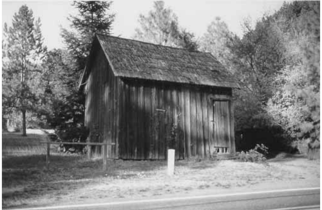
Figure 1.3.12 -Looking northeast toward the Golden Shed in a recent photograph, circa 2000 (GCW archives). Often referred to as a granary, the building's box construction suggests other uses.
