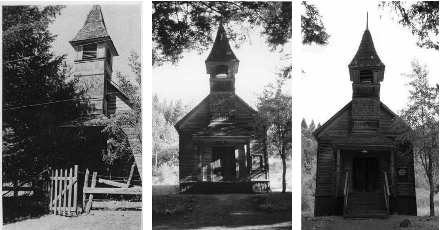
Figure 1.6.1 -Three views of the church: circa 1940 (left, GCW archives), circa 1990 (center, GCW archives) and 2007 with new porch (right, author's collection)
