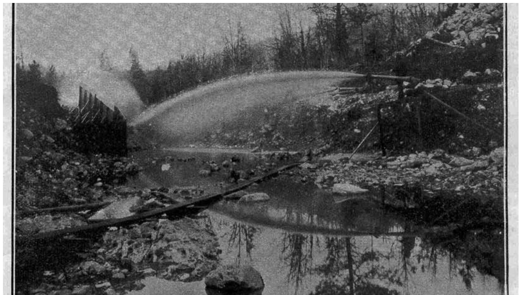
Figure 1.2.2 - A hydraulic giant sprays gold bearing alluvial soil into a Ruble Rock Elevator, circa 1900. By 1870, hydraulic mining was spreading throughout southern Oregon's placers (GCW archives)
