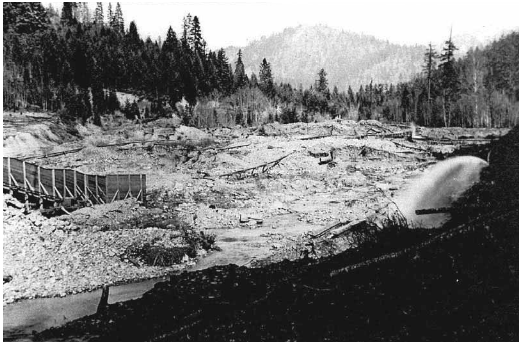
Figure 1.3.15 -Looking eastward up Coyote Creek near the settlement of Golden, circa 1900 (GCW archives). Note the extensive erosion of the Ruble's hydraulic mining activity, their elevator to the left, a giant to the right, a flume in the middle and a building (mining equipment shed?) near the flume.
