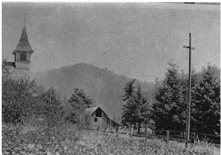
Figure 1.3.10 - Looking southeast toward Golden's church with the barn on the south side of Coyote Creek Road in the background, circa 1905 (GCW archives). William N. Ruble's large garden/agricultural field appears in the foreground. Note the power pole on the right edge of the photo and the orchard trees along the west elevation of the church.
