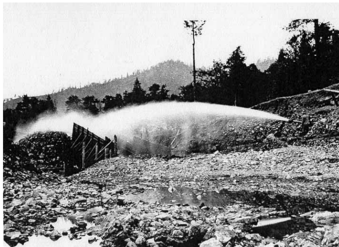
Figure 1.1.2 - Hydraulic mining with a Ruble Rock Elevator on Coyote Creek, circa 1900 (GCW archives)
