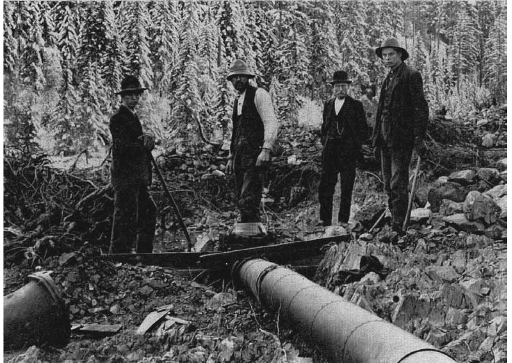
Figure 1.3.14 -Members of the McIntosh family inspect a blown waterline near Coyote Creek, circa 1900 (GCW archives). Such waterlines were used to feed the water canons, or hydraulic giants that blasted away up to 3,000 cubic yards of gravel per day.
