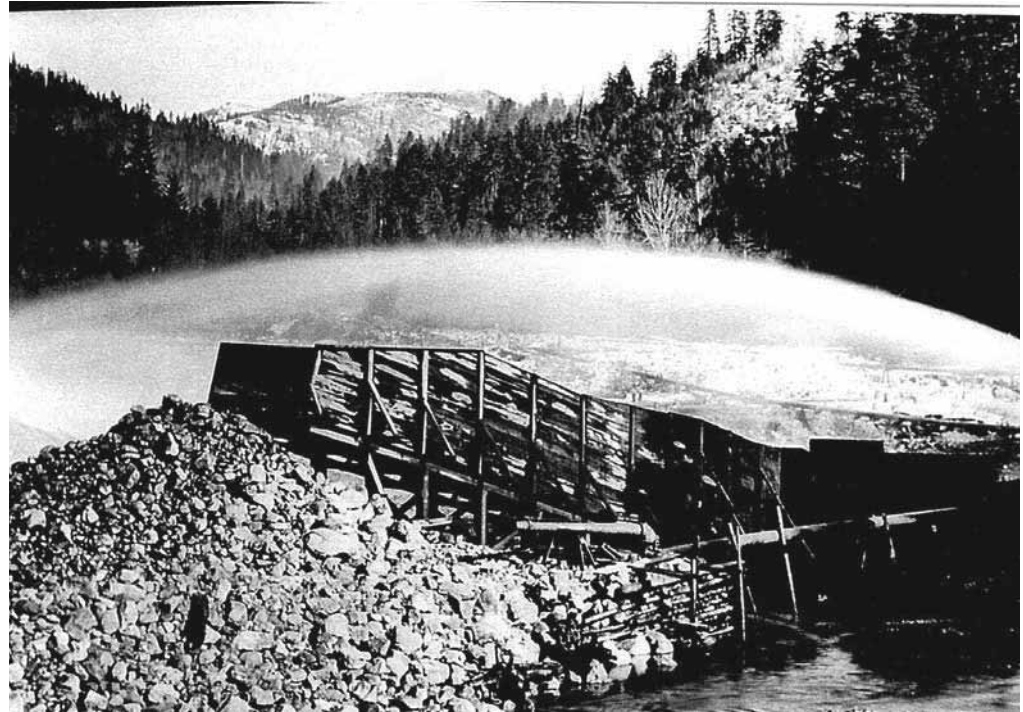
Figure 1.3.1 - Mining on Coyote Creek with a Ruble Rock Elevator and hydraulic giant, circa 1900 (GCW archives)
