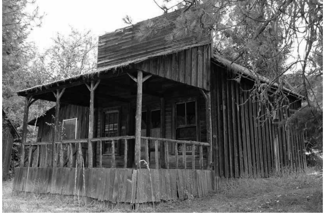
Figure 1.5.3 -Looking northwest at the Bennett's store in 2007 (author's collection). It is probable that Harry Aldrich replaced the front porch during the time he owned the settlement. Note the similarities in construction between the new porch and the stage below that also appeared during this era.
