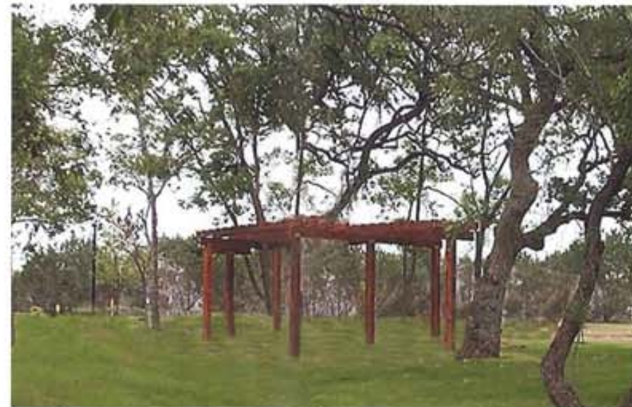
Sun shade shelters (example above) can provide a resting area for visitors to view the site. They will be built on the footprint of former structures, highlighting the extent and form of the old mining town.
