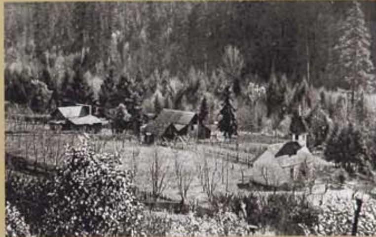
The community store (top left building) was located along the high street and supplied miners with all their needs, circa 1905 (GCW Archives).
