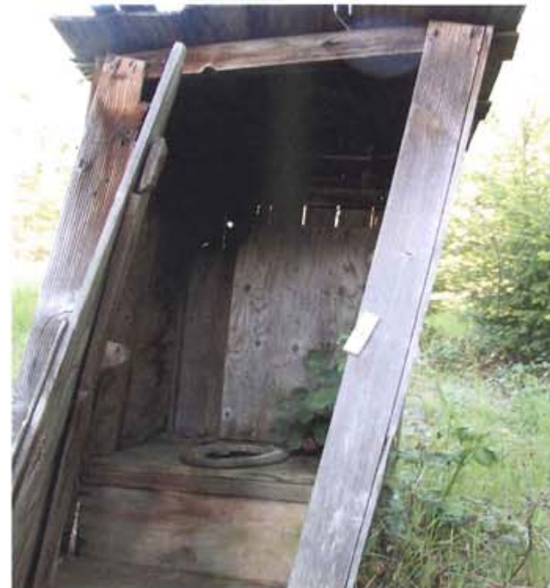
View of leaning outhouse adjacent to general store.
