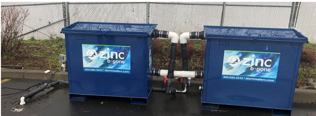
Second stormwater treatment system (zinc b-gone)
