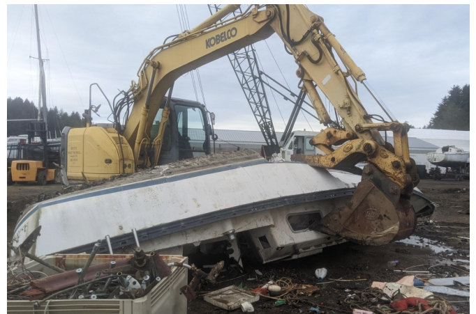
The final project was with the Port of Newport and was completed in June 2022.
