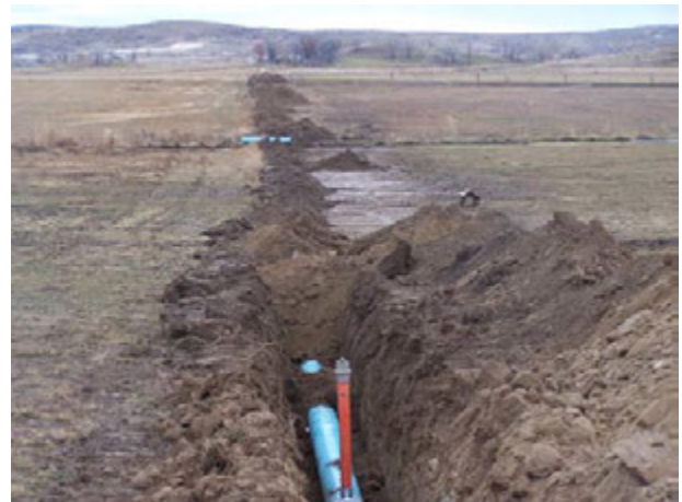
After: 2,800 feet of buried mainline for sprinklers.
