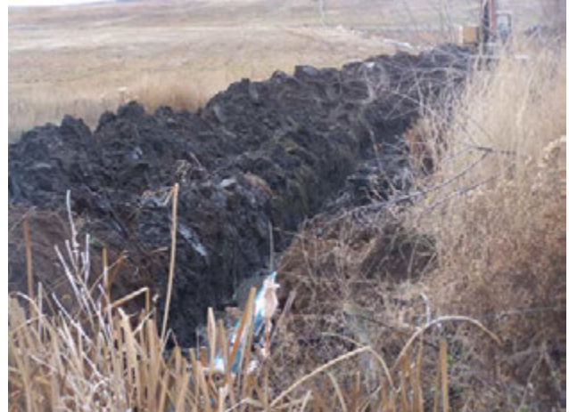
After: water will now be captured in this pipeline being installed and bypass the feedlot.
