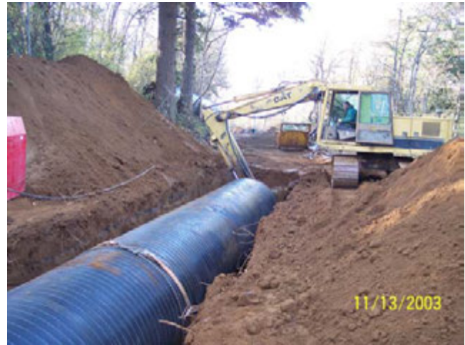
Figure 2. EFID CLPP “Upper Phase” work in 2003 ( new system ).
