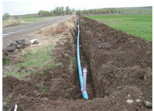
After: 2,700 feet of buried mainline and sprinklers.
