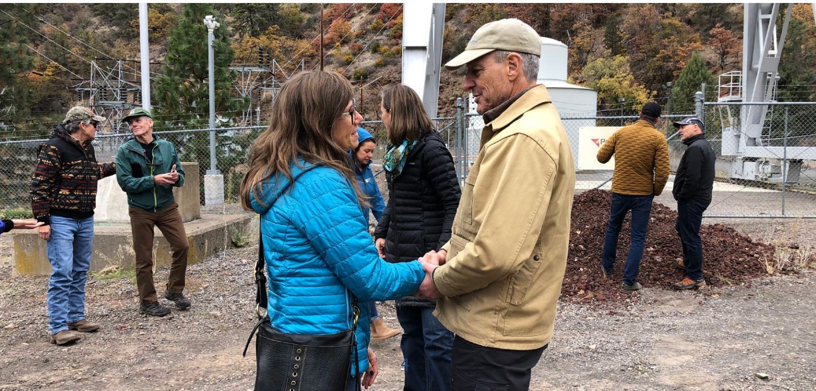
OWEB met with partners at the JC Boyle Dam removal site in October 2023.
