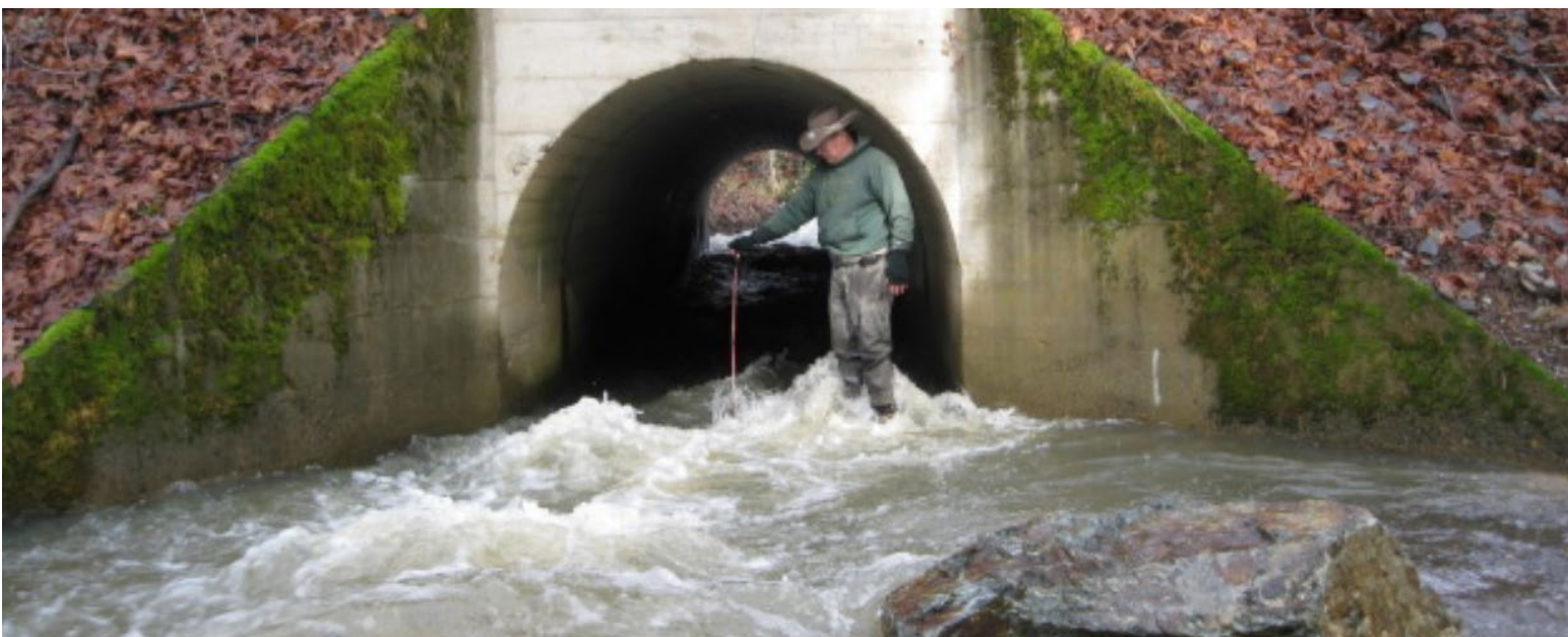
Railroad culvert on Jones Creek after passage project.
