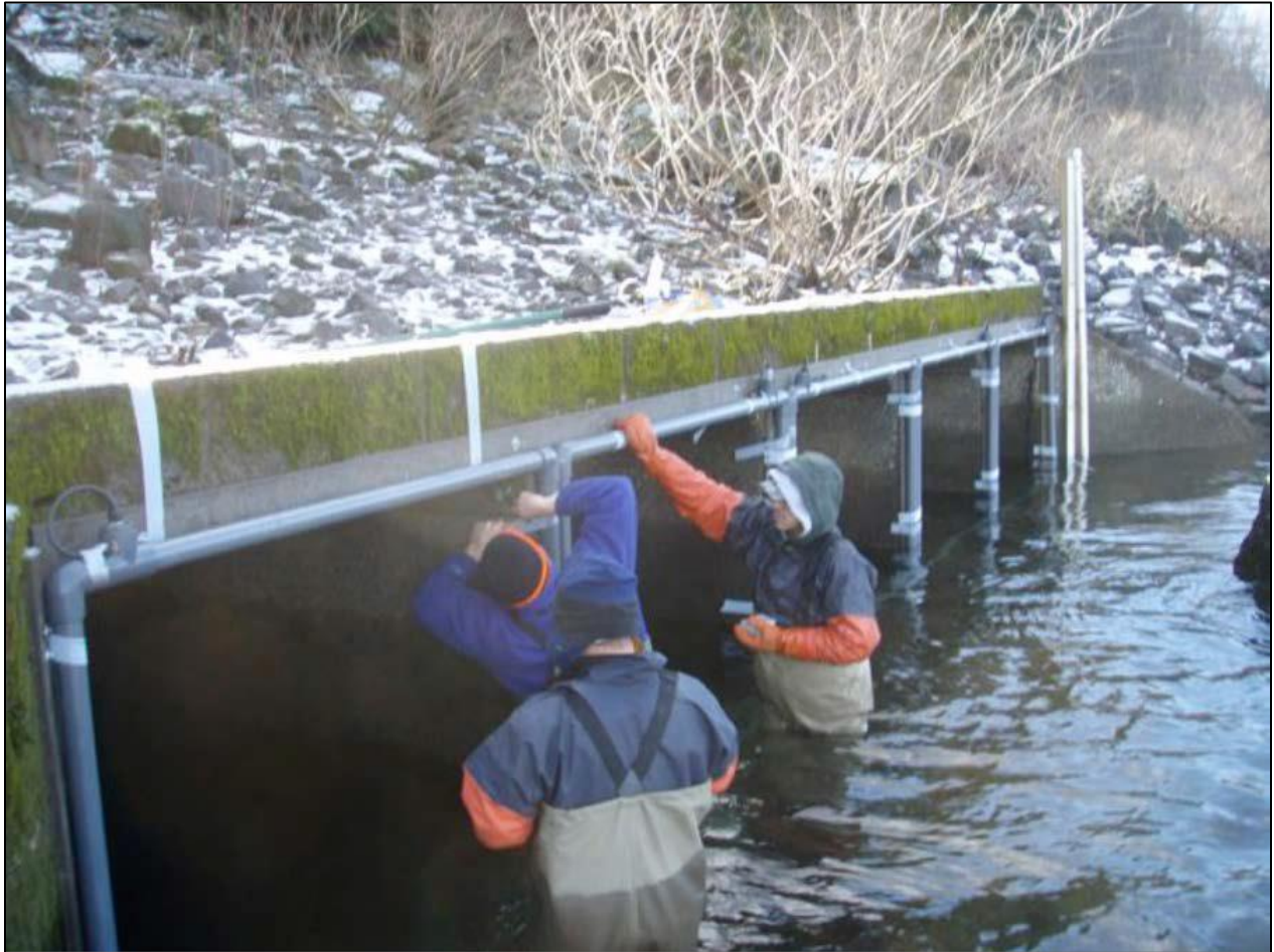
Figure 8: Downstream side of PIT tag array at Horsetail/Oneonta creeks outlet culvert.
