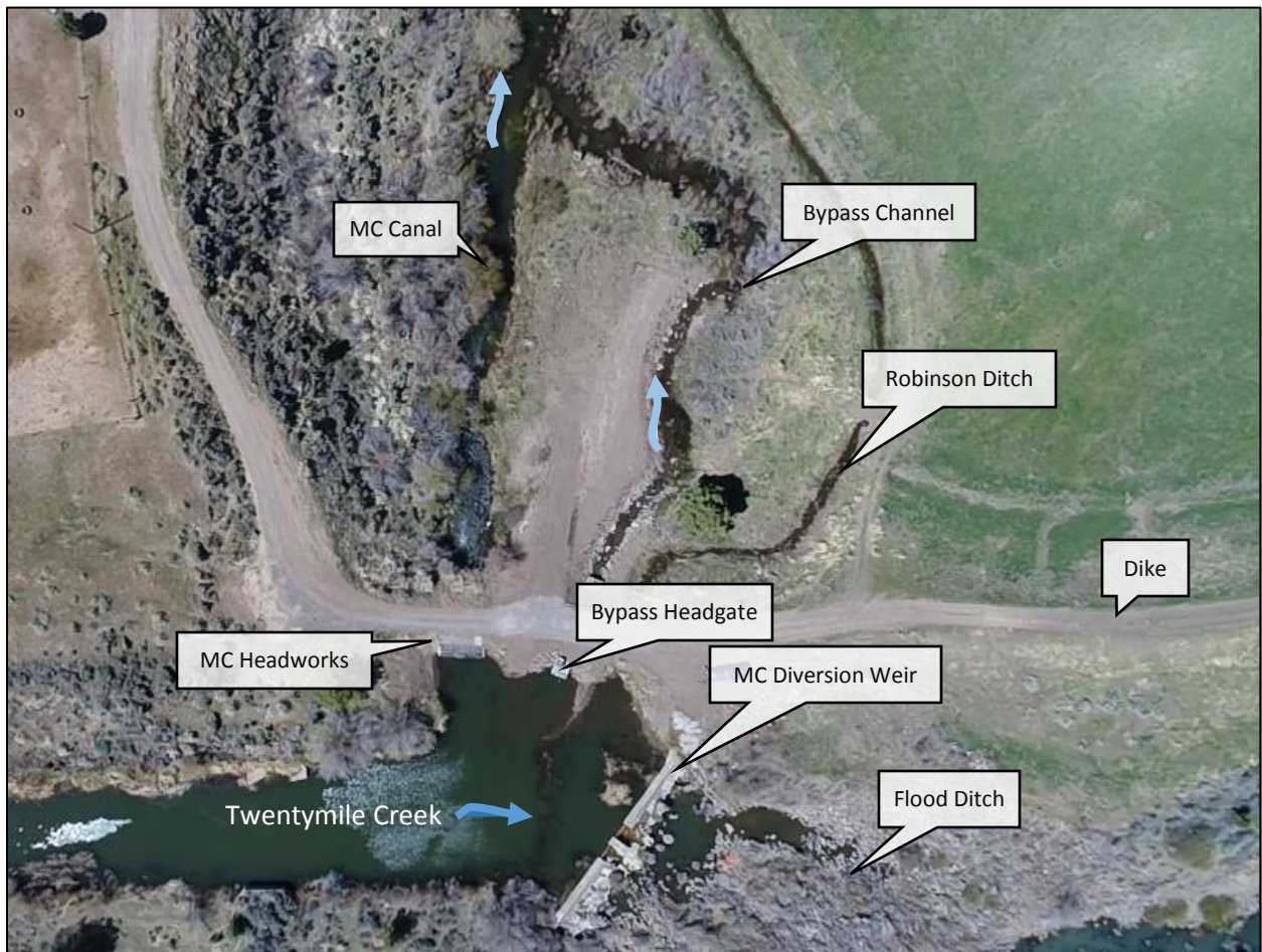
Figure 6-6. Low elevation aerial photo showing the MC diversion area features.
