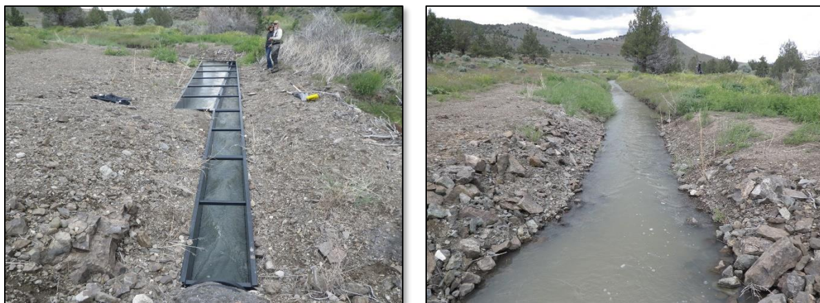
Figure 6-3. The FCA fish screen on the Dyke diversion irrigation canal (left) and the open canal downstream of the screen (right).
