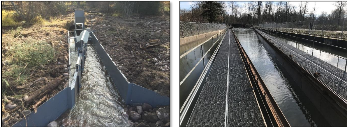
Figure 5-7. Example vertical flat plate screens in single (left) and double or “vee” orientation (right). Screens are actively cleaned by powered brush systems.
