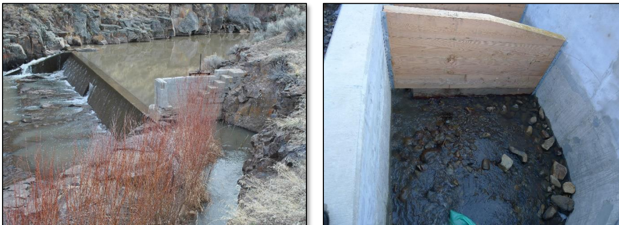
Figure 6-1. The existing Dyke diversion weir showing the weir, Denil fish ladder, and headwall with irrigation canal (left). The fish ladder completed in 2015, includes wooden weir walls with a 12-inch square orifice and streambed simulation material (right, photo during construction).
