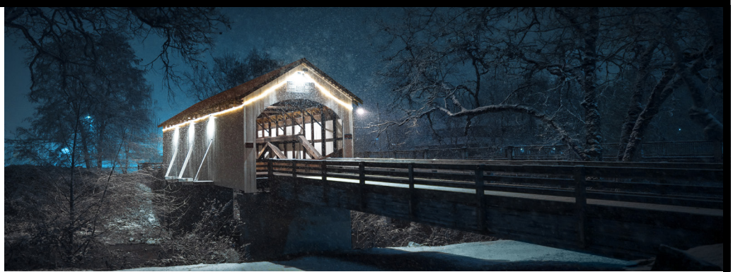
Antelope Creek Bridge, Eagle Point, Oregon
