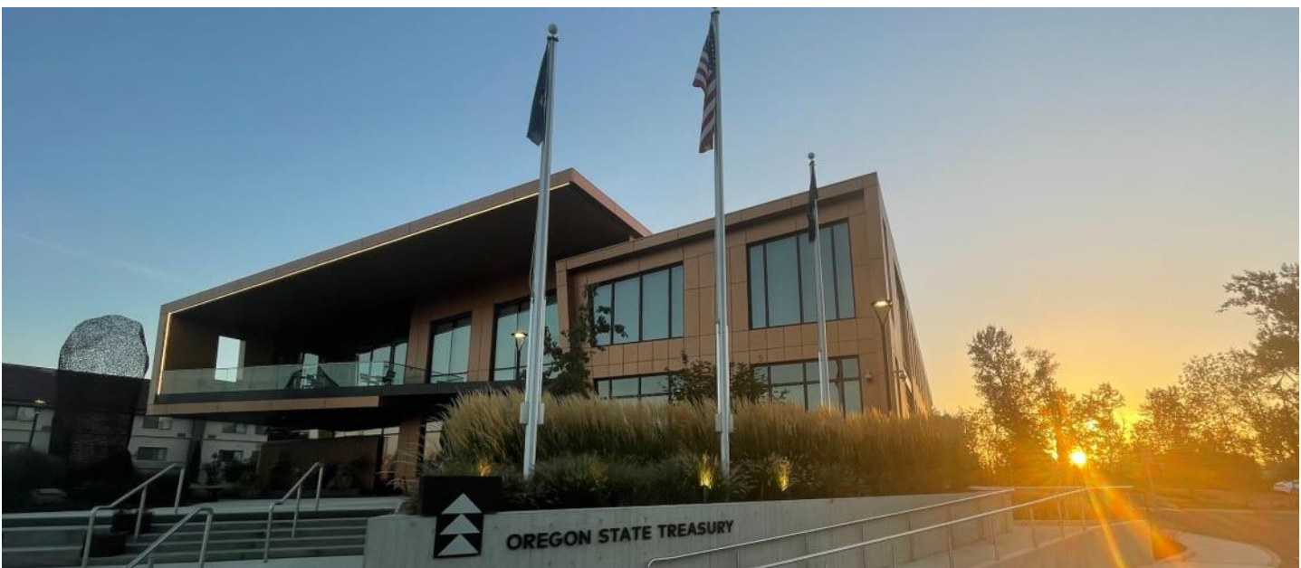
Treasury’s Mill Creek Resiliency Building in Salem was designed to ensure the state’s financial business is not disrupted following an earthquake or other disaster.
