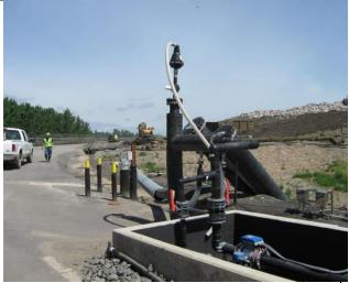
5. Leachate collection piping controls for Module 9. Air relief valve had been releasing some leachate, so hose was connected to direct this liquid to the concrete containment area. WM notes they are working to repair this. Leachate collecting in this containment structure drains to the leachate collection pond.
