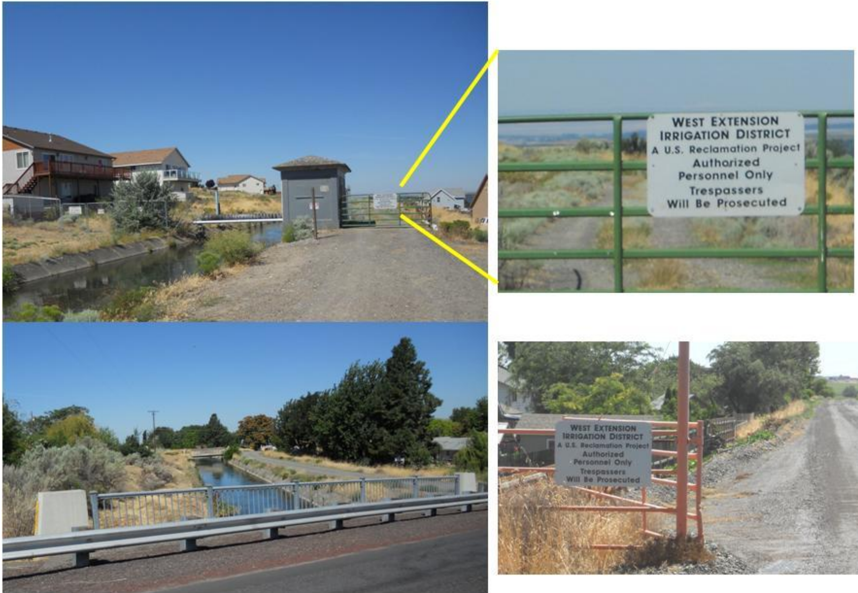
Figure 10. View of Canal signage and access controls, from the canal bridge crossing at Umatilla, Oregon
