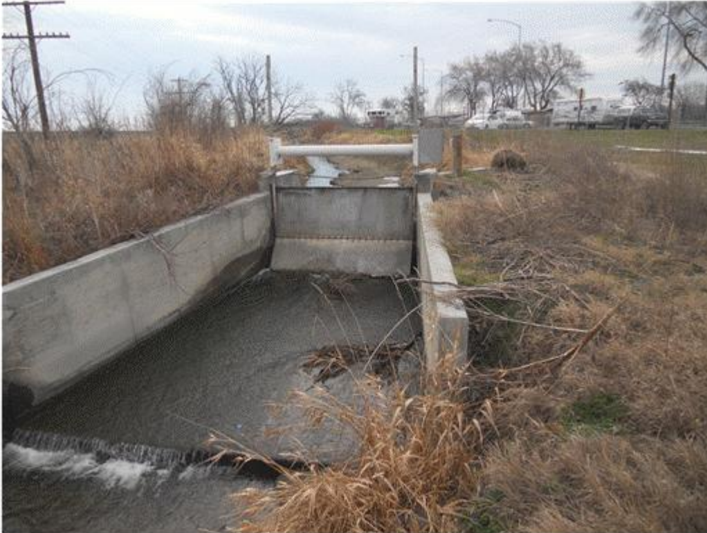
Figure 8. Fish Barrier near end of canal overflow channel (2011 photo) (Boardman Interstate-84 Rest Area is visible in background)
