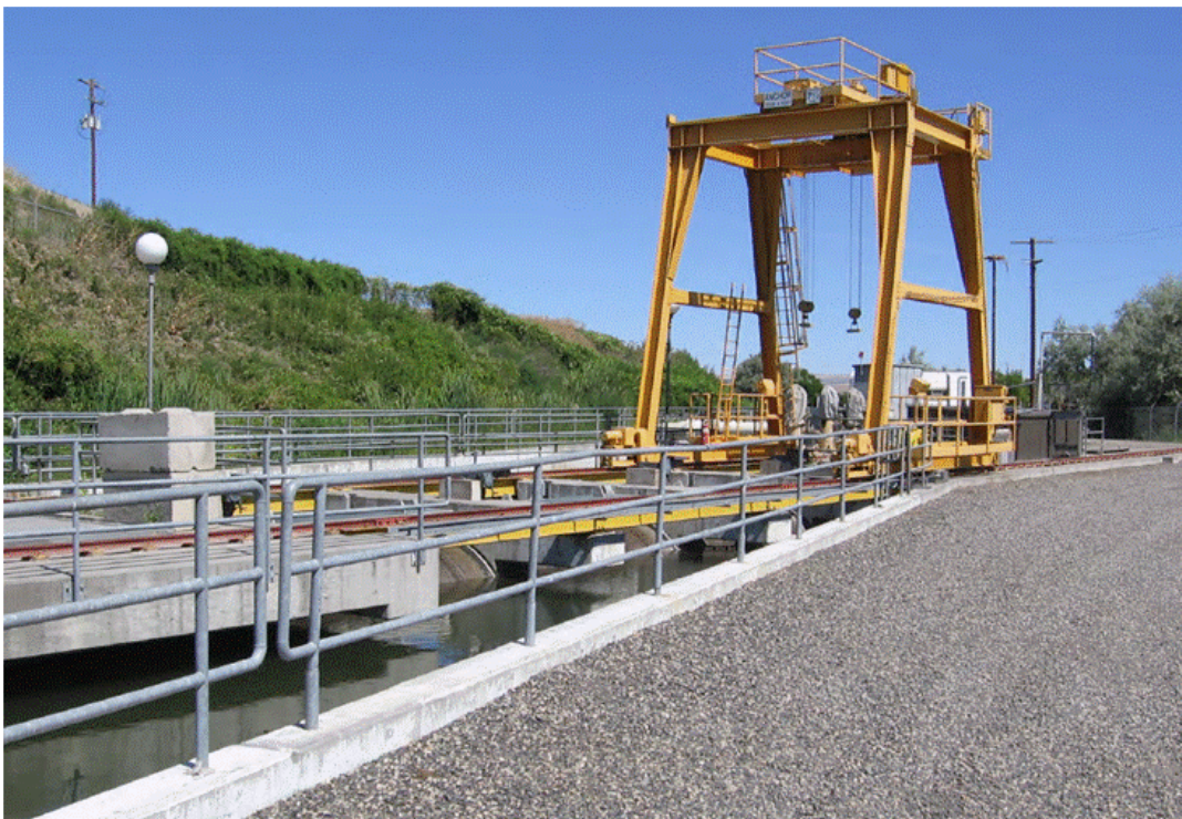
Figure 7. Fish screen at Three-Mile Falls Dam (OWRD website)
