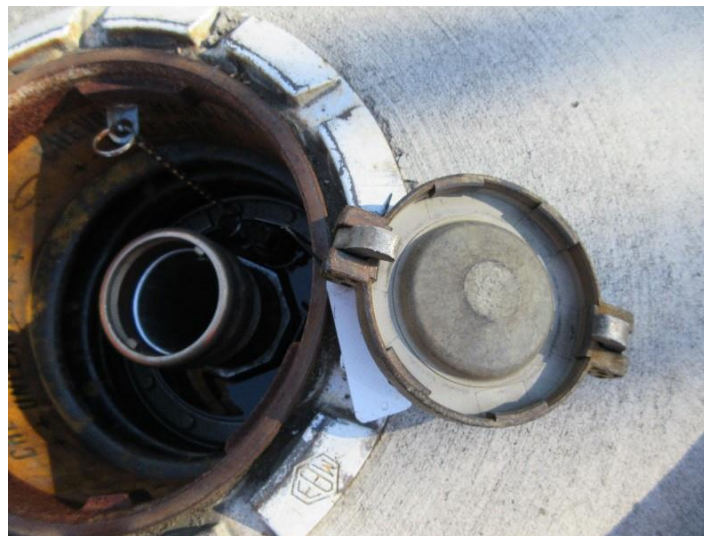
Dust Cap/Fill Tube- No gasket seal.
