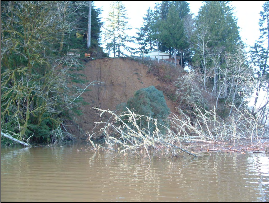
Figure 39 – Lakefront Development Slope Failure
