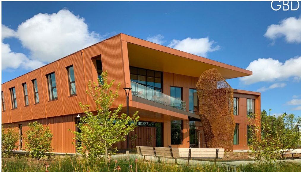
Figure 1. The Mill Creek Resiliency building is the first United States Resiliency Council Platinum-rated structure in Oregon and first building made seismically stable as a base isolated structure in the United States. Photo credit: GBD Architects.
