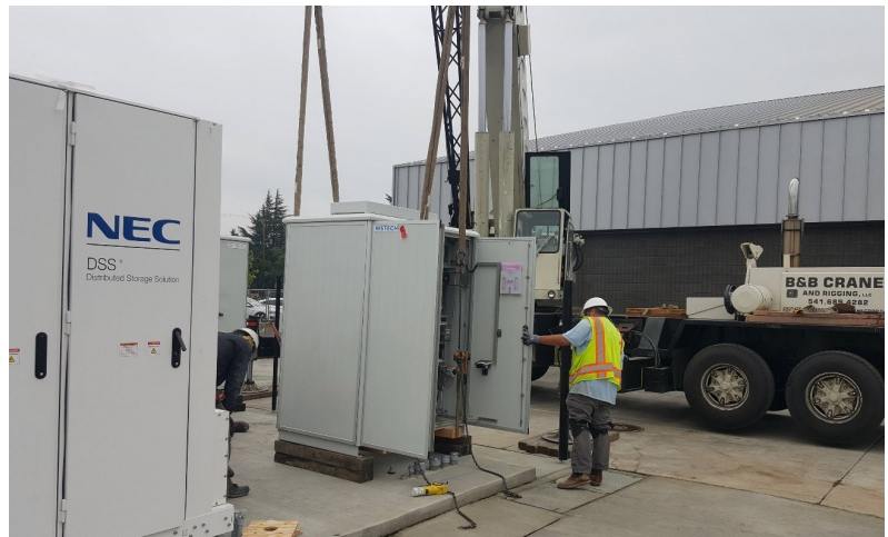
EWEB contractor installs back-up battery power system.
